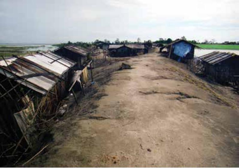
Human settlements built close to embankments are a major cause of deterioration
